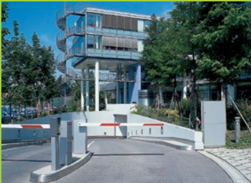
Our aesthetic solutions for traffic areas, Landeszentralbank in Munich.
